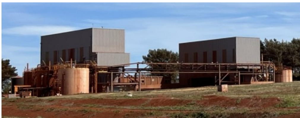
Figure 6. Press filters in Mange Garri bauxite residue storage facilities.
